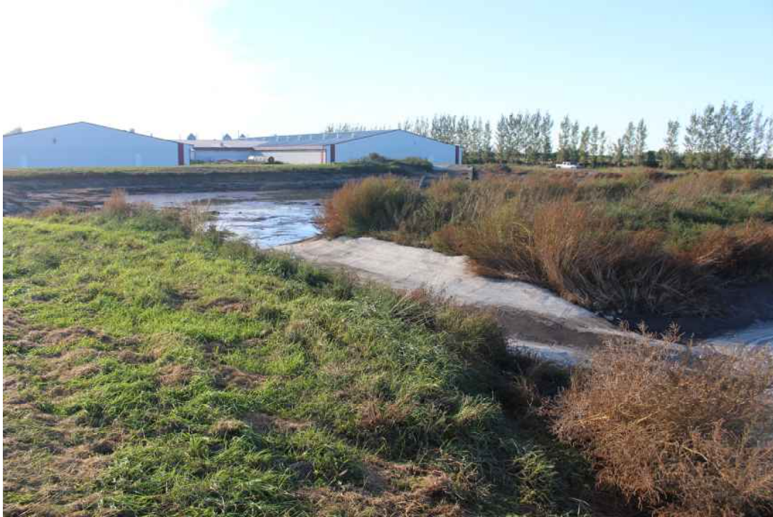
Cross over channel between primary and secondary cell at first and third strategy
